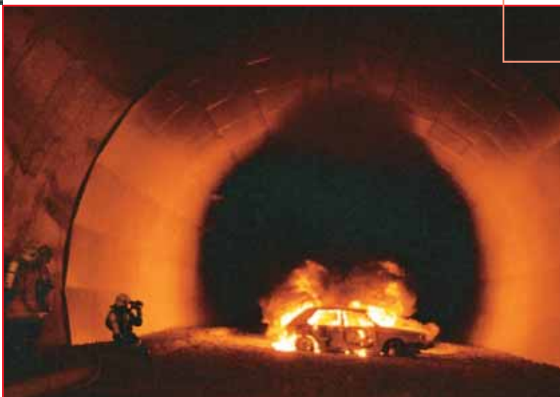
Tunnel des Bruyères, fire drill; structural concrete protected with AESTUVER dicon tu fire-resistant boards in test area
