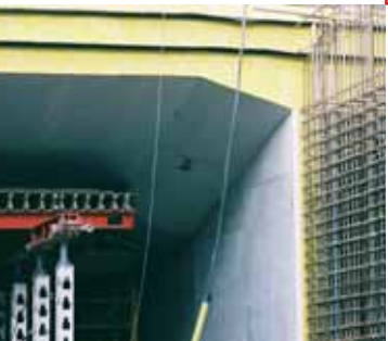
Lilla Bommen Tunnel, Gothenburg, Sweden; dicon tu, 30 mm, set in concrete; system tested with HC curve; 180 minutes plus
