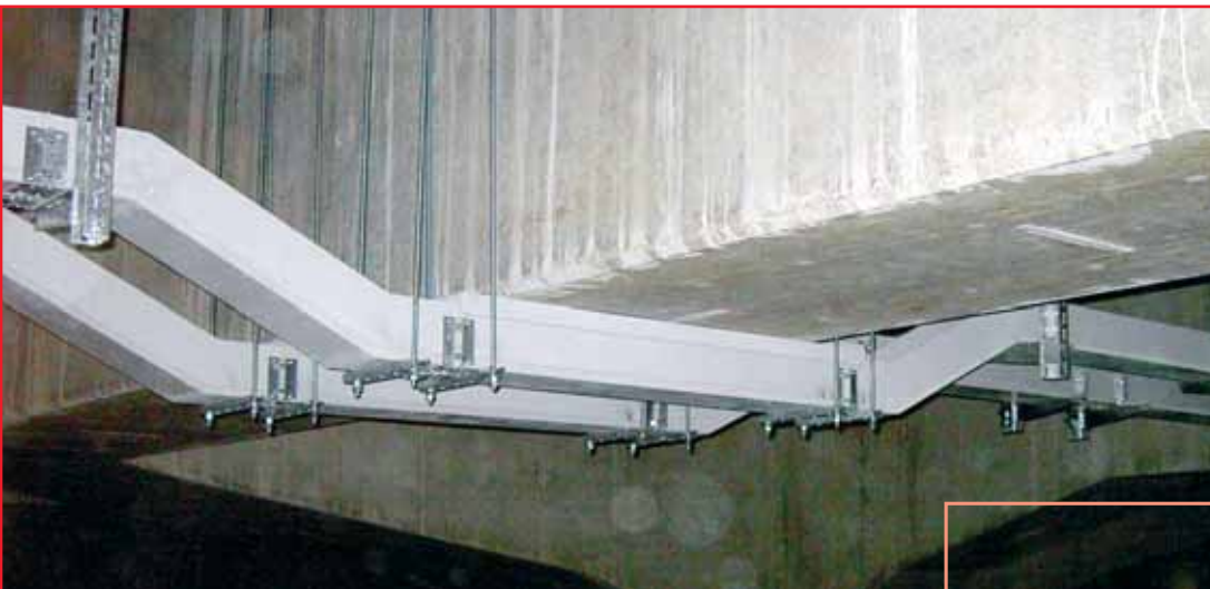
Suspended AESTUVER fire-resistant cable ducts
