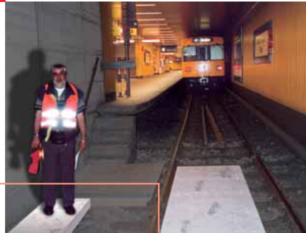
Berlin underground railway; covering for timber sleepers
