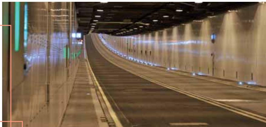
2 nd Elbe tunnel tube Hamburg
