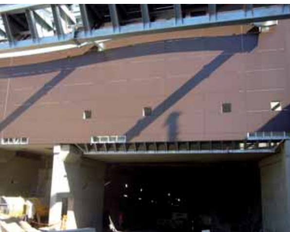
NSBP tunnel Brisbane
