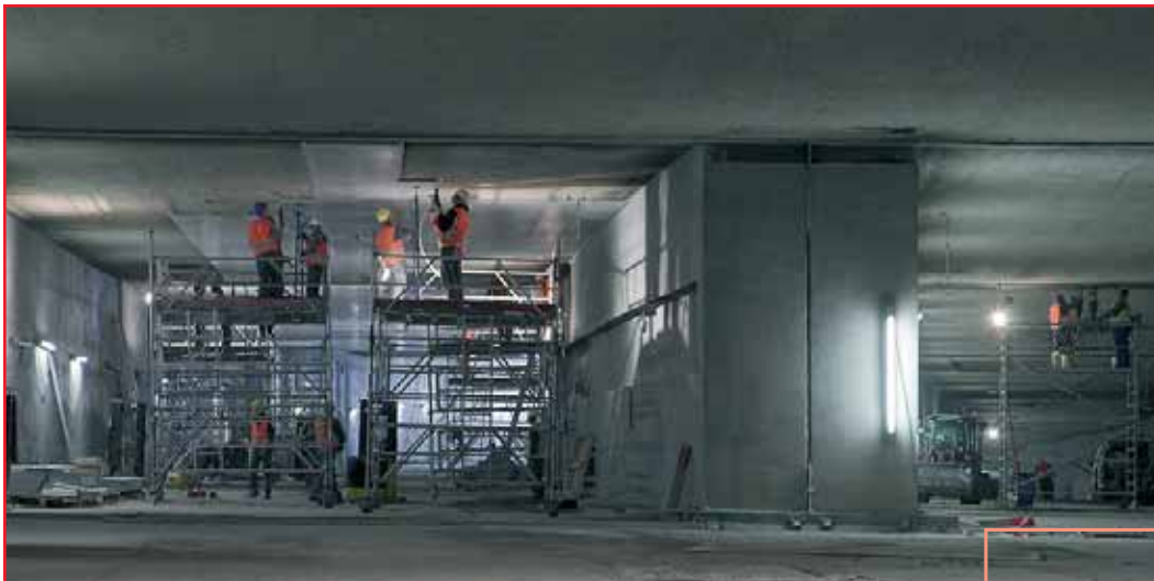
Berlin Tegel airport tunnel
