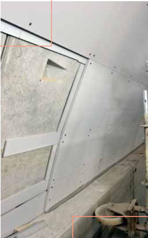
Joint with joint backing strips
